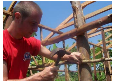
Paul Robinson helps with nailing the fitos to the posts
